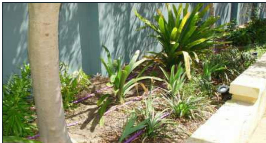
Purple drip irrigation lines are used to indicate greywater reuse in residential gardens.
