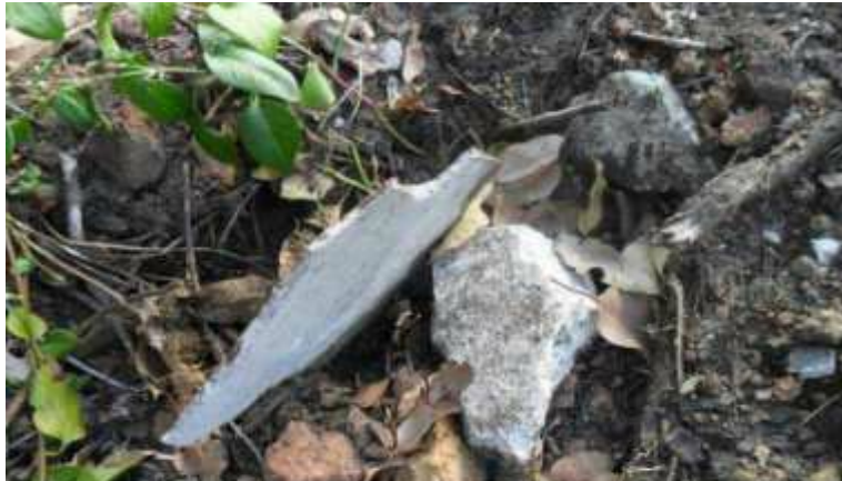
Asbestos contamination detected during a site investigation
