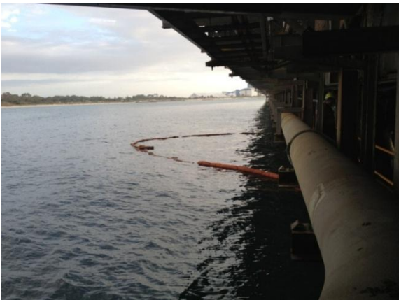
Figure 9 Diesel spill into Cockburn Sound. A bund was placed around the Coogee chemical pipeline fissure. Source DER
