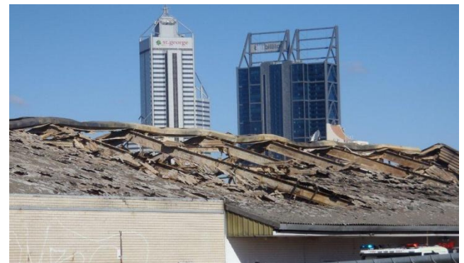
Figure 3 Asbestos roof burnt during a fire in Northbridge
