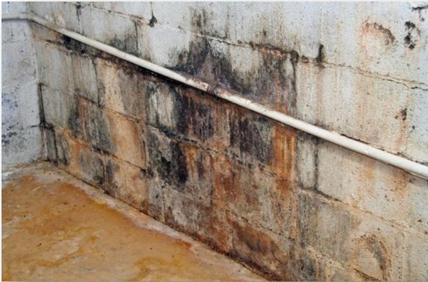
Figure 5 Mould damaged building
