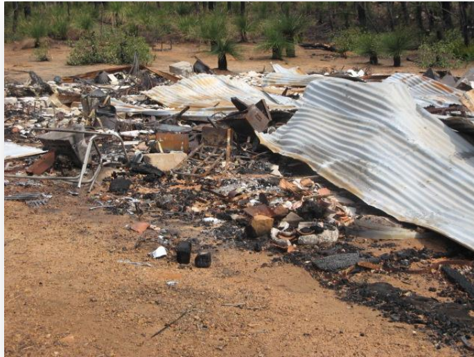
Figure 1 Asbestos contamination following the 2011 Margaret River bushfires
